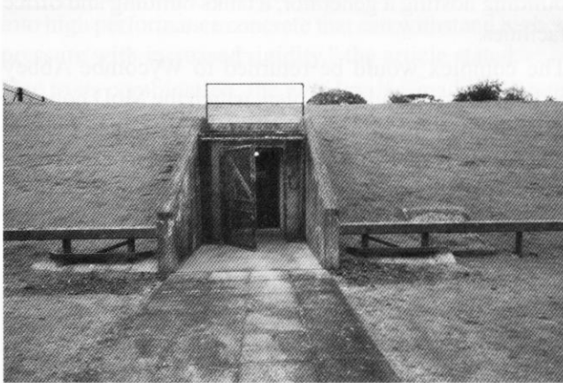
Main entrance to the Ballymena RGHQ. Photo Nick Catford
